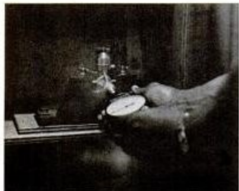
Handy with lathe (right above), Stockton modified standard Eta engine into heavier, more reliable one held in his right hand (top left). Above left, he times engine's 15,200 rpm.
